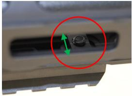
**4.1.4** The M-LOK<sup>TM</sup> rail may not fit in the bottom two, forward-most square slots on the FN15<sup>TM</sup> Tactical Carbine because the gas block will interfere with the locking pieces of the rail. Additional M-LOK<sup>TM</sup> rails and accessories are available directly from Magpul®. (www.magpul.com)
